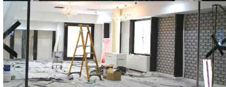
Coffs Central Stage 1 (Photo: Oct 2012)
